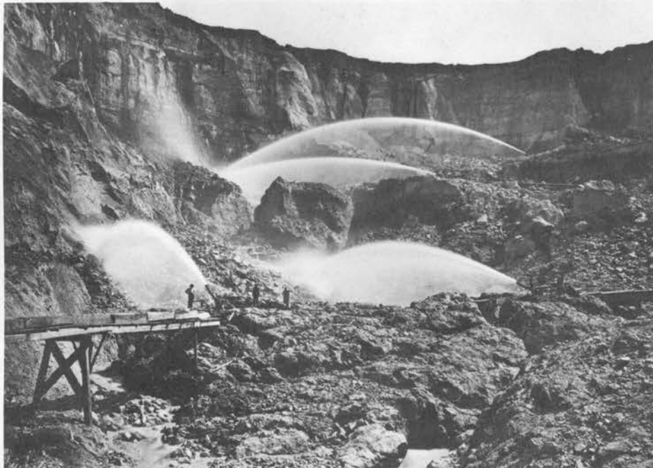
Hydraulic mining, Malakoff Diggins, Sierra foothills, by C.E. Watkins, 1871 Courtesy, Bancroft Library.
